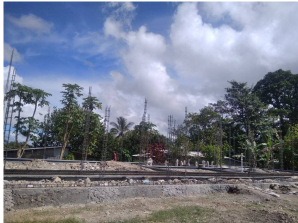
Foundations are laid for the new kindergarten
