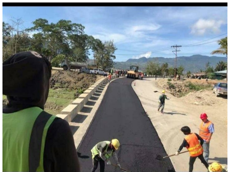
Road construction looks amazing on the Baucau to Venilale road
