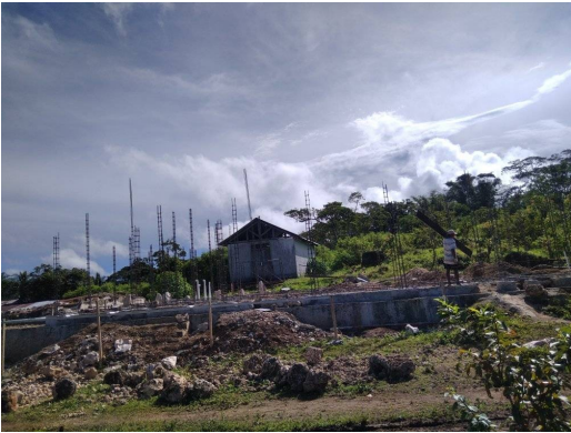
Uai Bua - the foundations are laid for the new staff room
